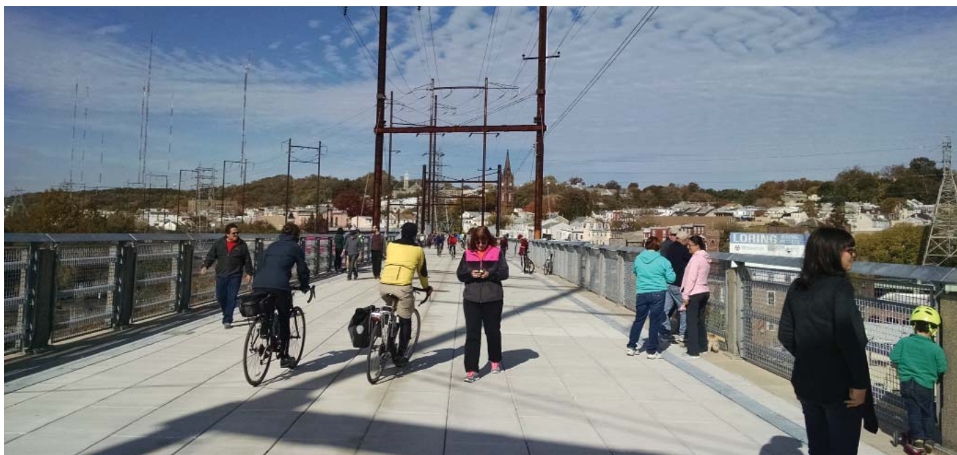
Completed Manayunk Bridge Trail
