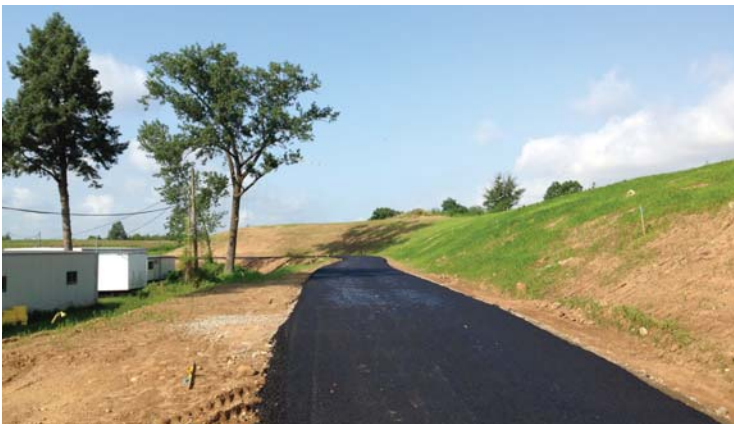
Baxter Trail Under Construction - Delaware River City Corporation
