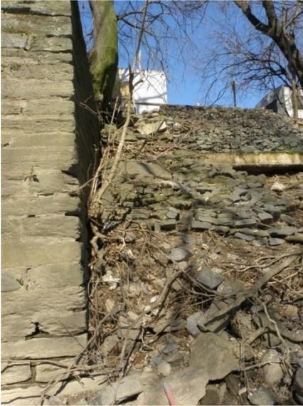
Undermined rock slope protection
