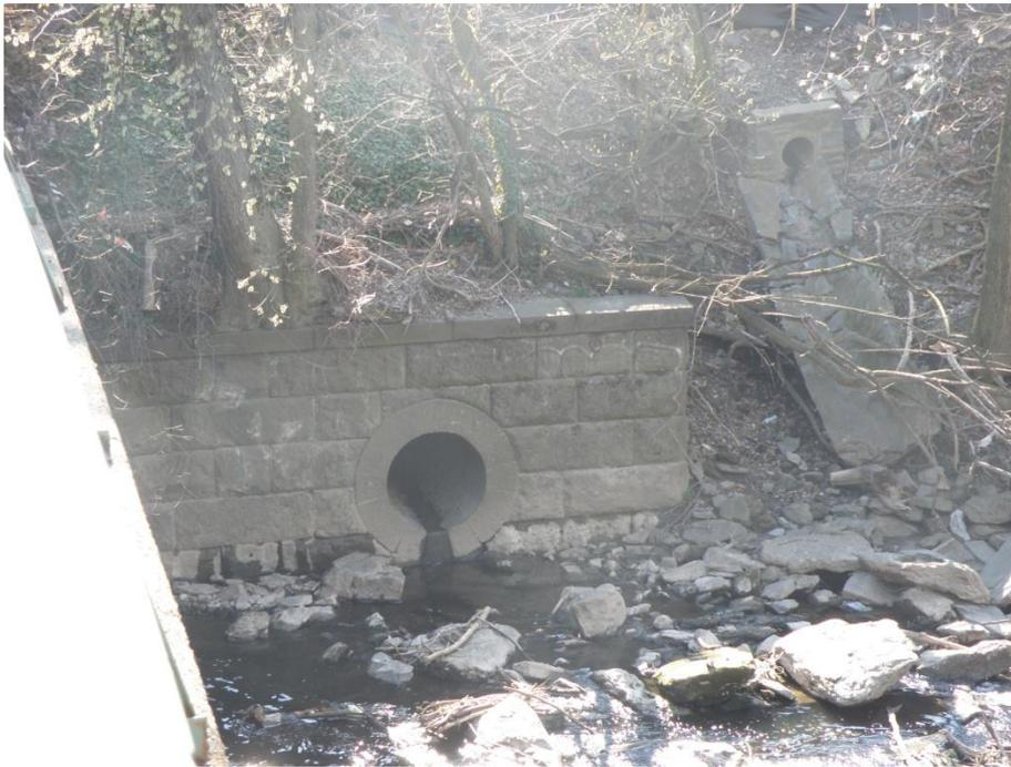
Construction of new abutment extensions would be expensive as the banks are steep and features above would either prohibit excavations or require extensive shoring. Post and panel wall would probably be the most economical alternative. Work in this location is probably the most costly alternative.
